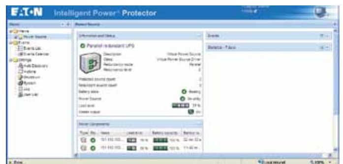
Support for redundant power
